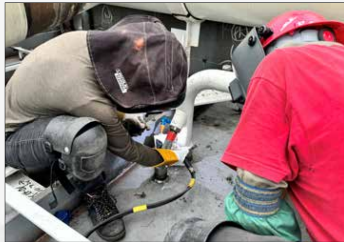
Shayla Baker , Pipe Welder and Jorge Luis Zavala-Godoy , Welder Trainee A
