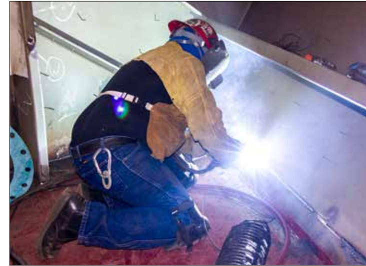
Israel Jimenez, Subcontractor, Production Welder, welds Hull with a hand-held gun
