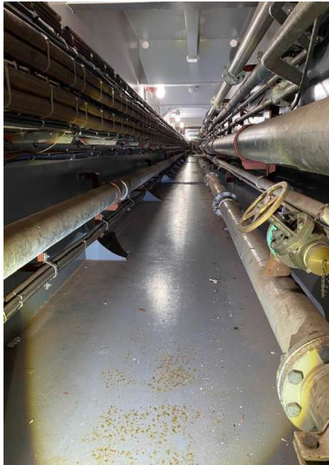
Photo 16 - Typical Condition of Crossover Tunnel
