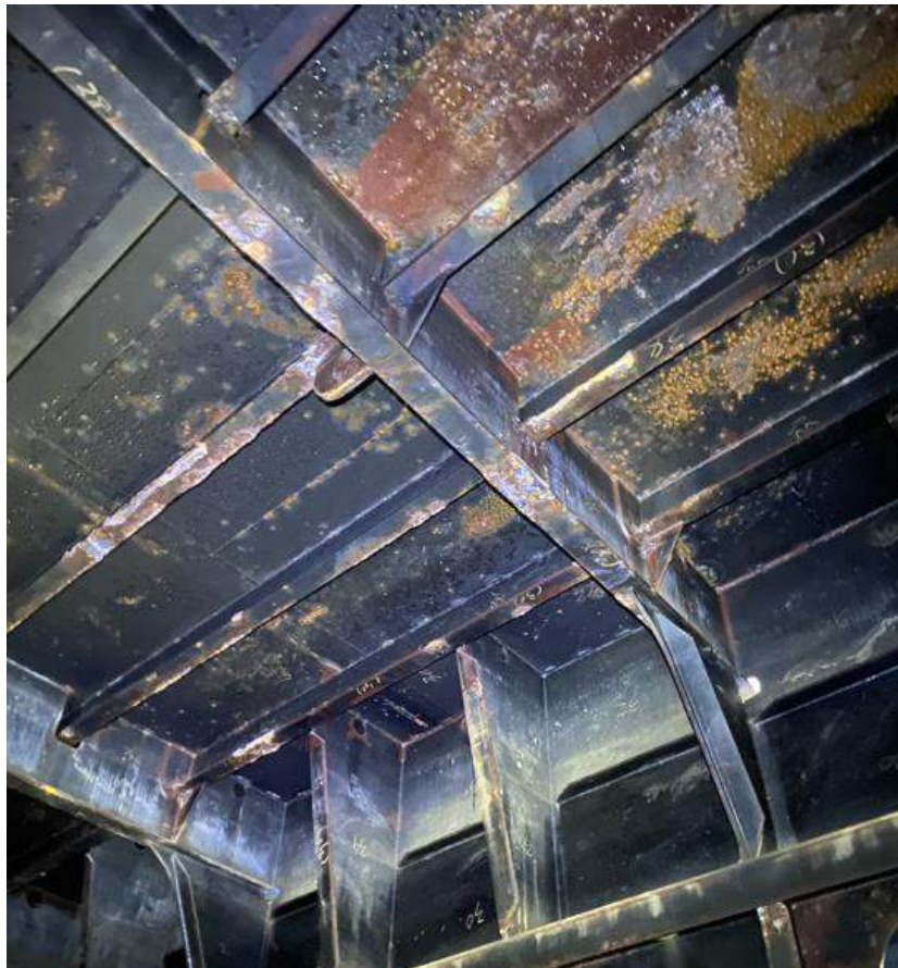
Photo 8 - Typical Condition of Wing Ballast Tank
