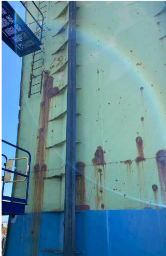
Photo 37 - Condition of 45 deg. Mooring Tee
