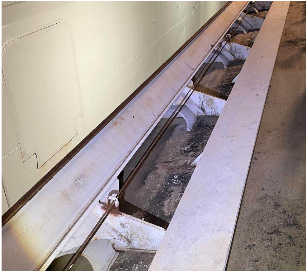
Photo 45 – Typical condition of trolley track
