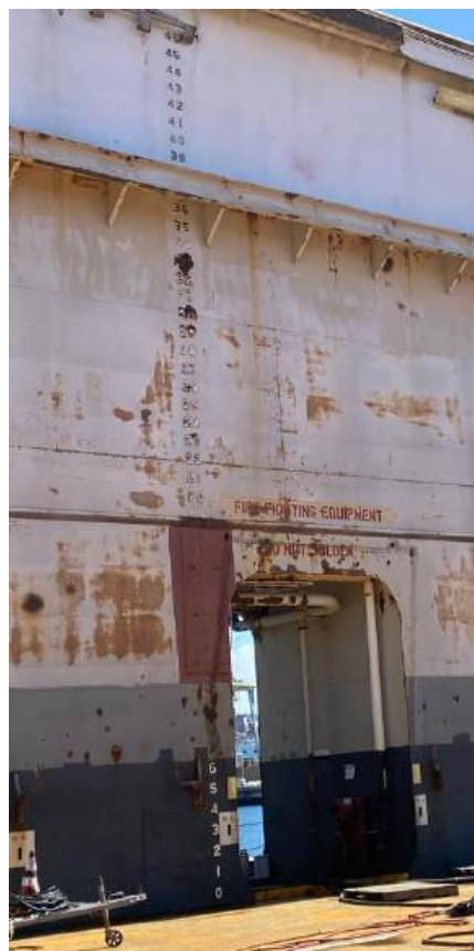
Photo 36 - Condition of Draft Boards Internal
