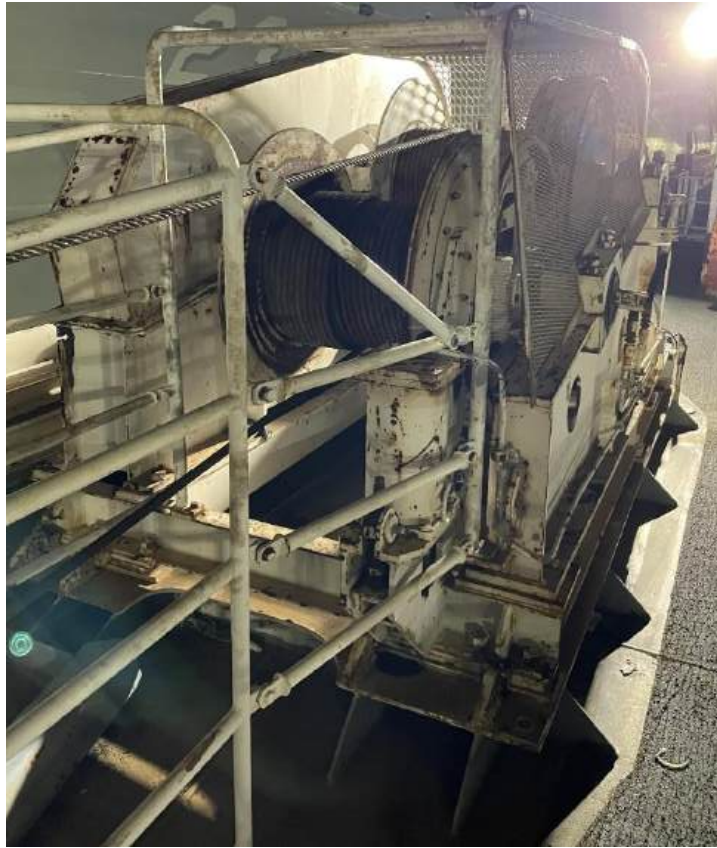
Photo 43 – Typical condition of vessel handling winch
