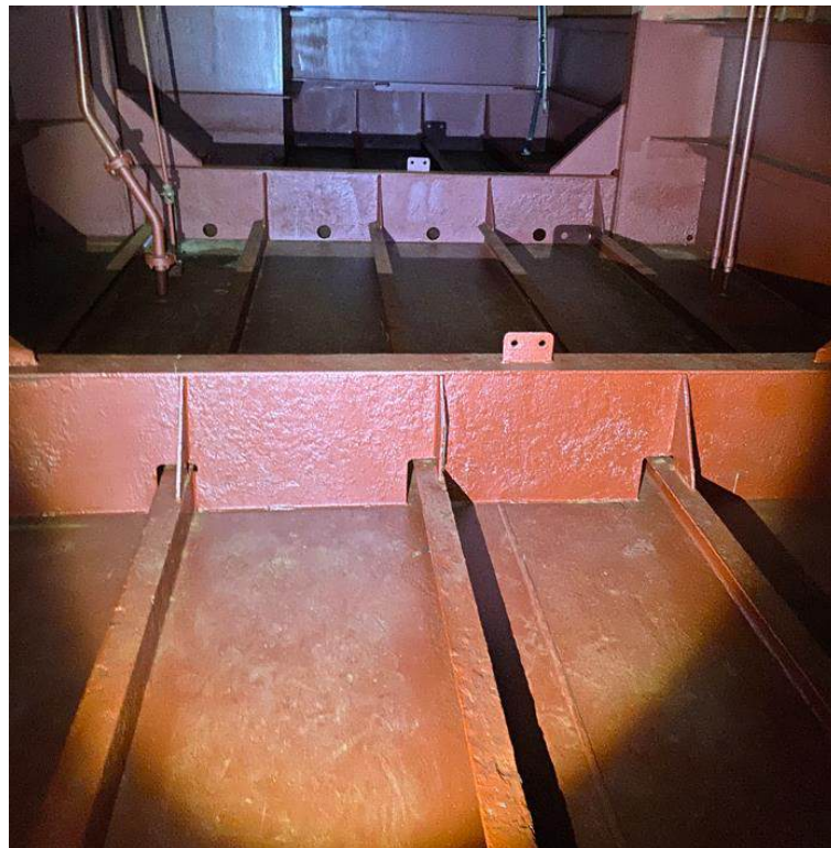
Photo 18 - Condition of Port Fwd-most Void
