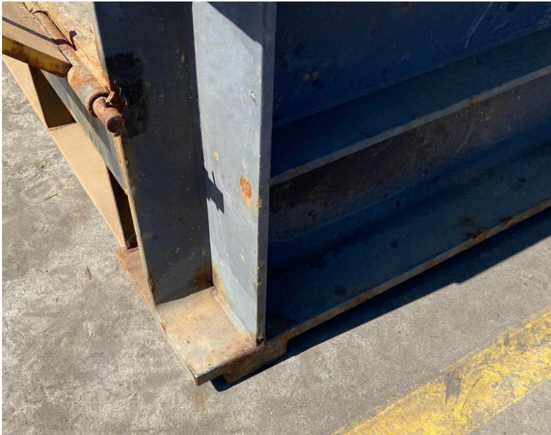
Photo 34 - Condition of Vehicle Ramp Structure and Bearing Pads
