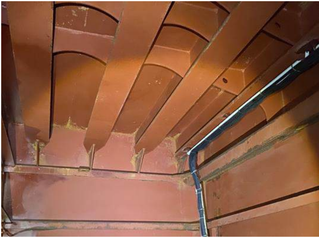
Photo 19 - Condition of Port Fwd-most Void
