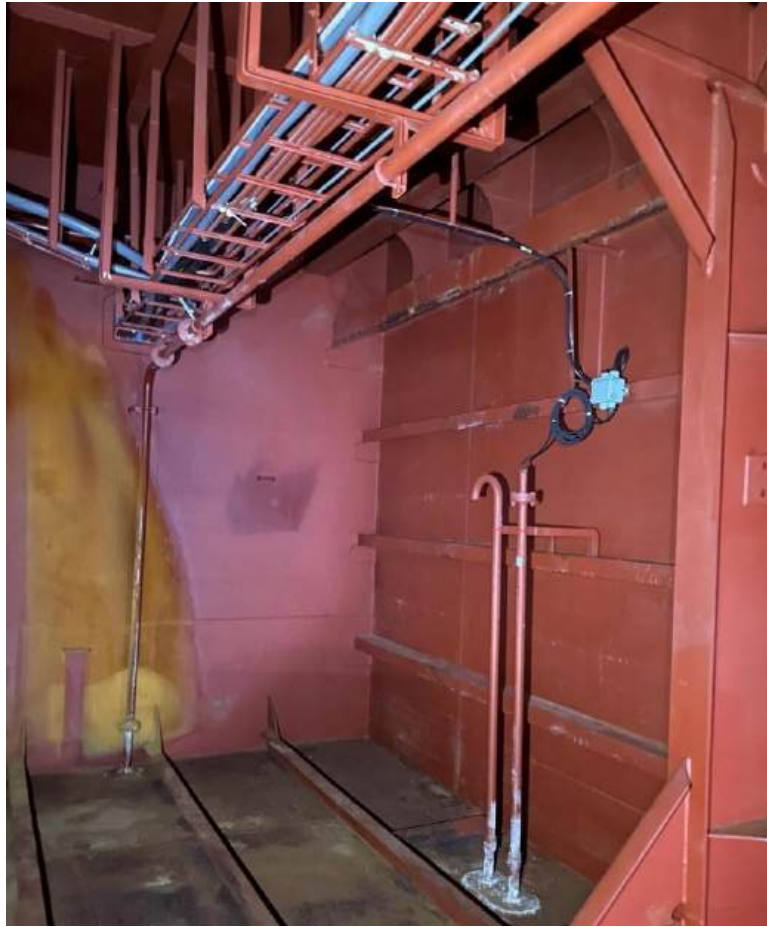
Photo 17 – Typical condition of port side void spaces
