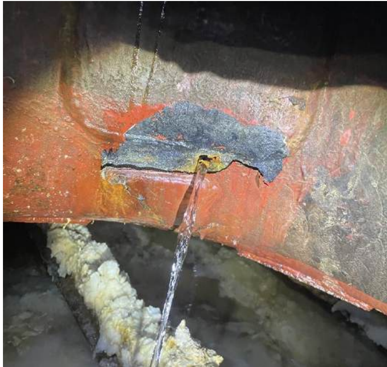
Photo 83 – Tank 4-S (FR 81): Discharge pipe has 1/2" diameter hole in doubler plate.
