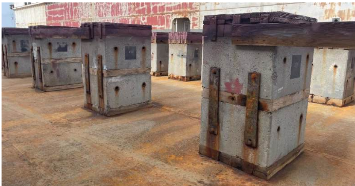
Photo 50 – Typical condition of keel and side blocks
