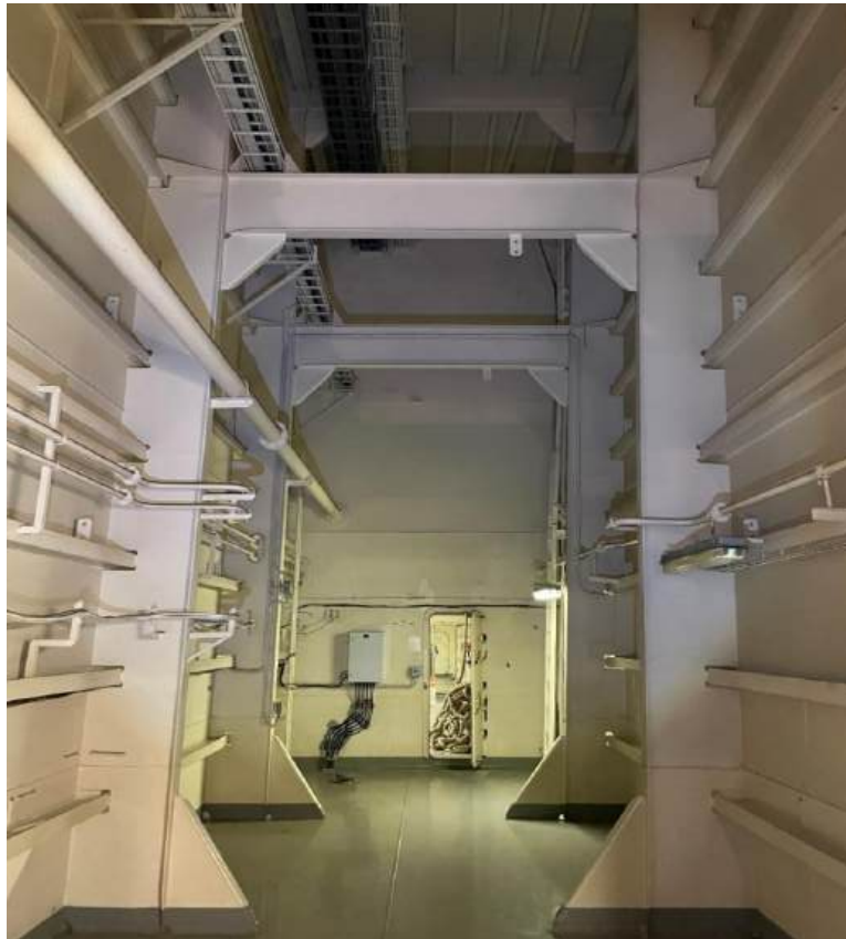
Photo 14 – Typical condition of safety deck (Port shown)
