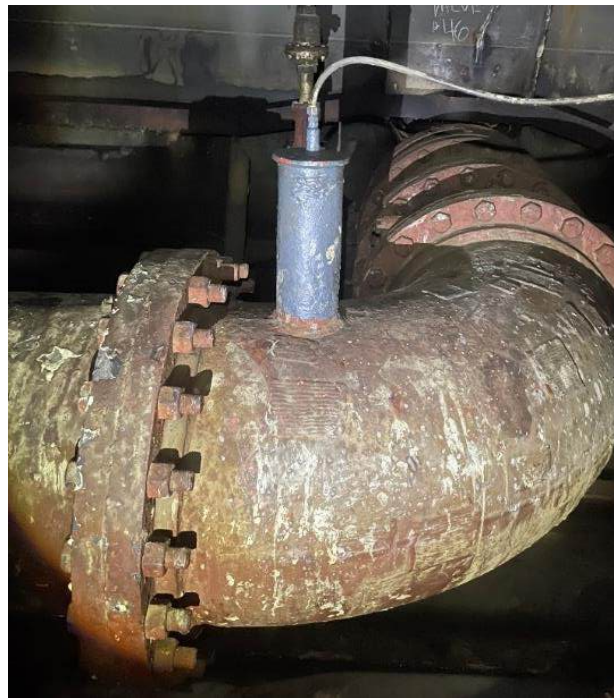
Photo 83 – Tank 4-S (FR 81): Discharge pipe has 1/2" diameter hole in doubler plate.
