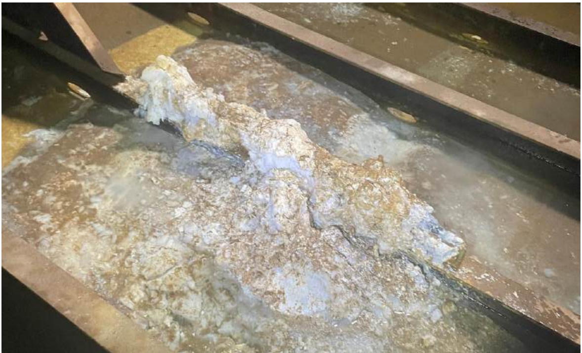
Photo 6 – Typical wasted anode in need of replacement
